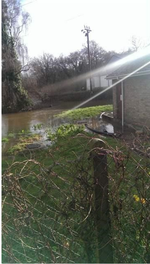
Wessex Water Pumping Station (Right of picture), viewed looking South
