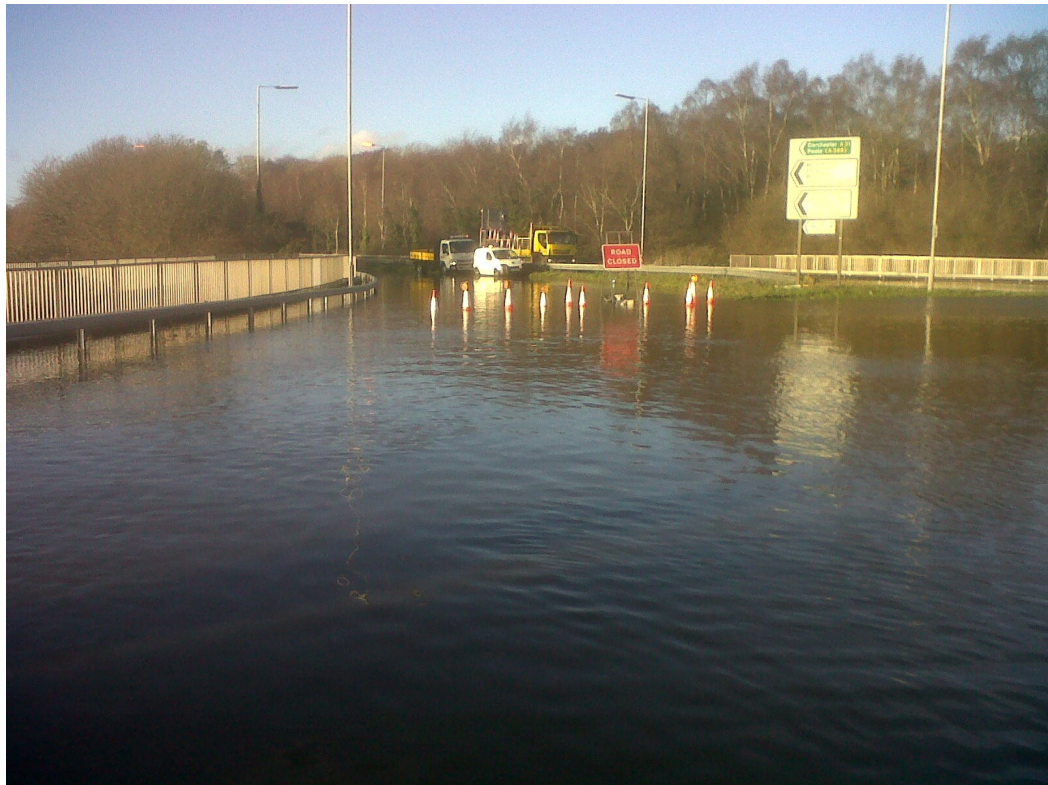
Palmersford Roundabout, viewed from dual carriageway, looking North West
