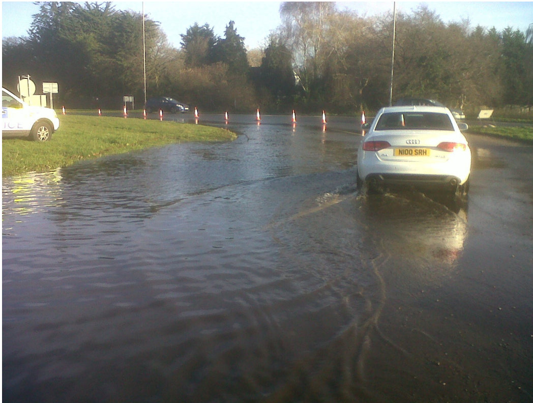
Palmersford Roundabout, viewed from dual carriageway, looking North East
