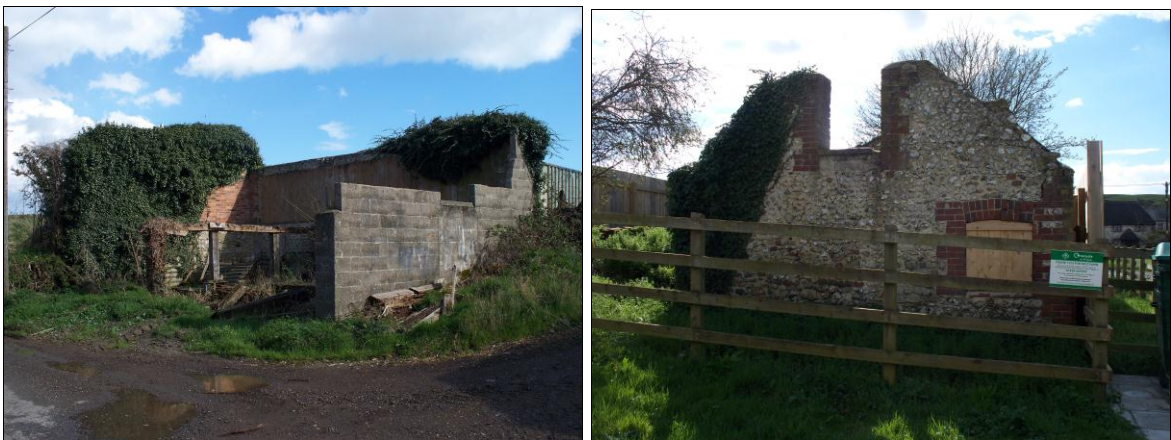
FIG. 13: Ruined buildings. Left: former agricultural building at Vicarage Farm. Right: the listed Old Forge on the green.
