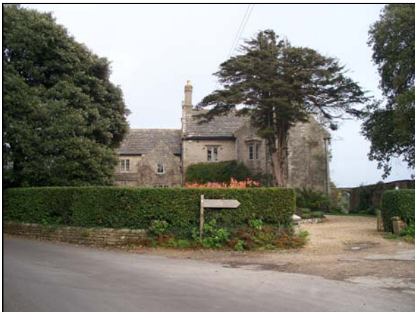
FIG. 9: The Old Rectory. Stands prominently closing the vista at the east end of the main street. An interesting neo-Gothic exercise in the Purbeck stone vernacular.
