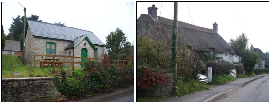
FIG. 10: Roofs. Left: slated roof of the Reading Room, typical of nineteenth century development in Church Knowle. Right: thatched roof of the Old Cottage more typical of earlier properties. Note the traditional flush ridge. Block ridges have been introduced to all other thatched properties here.
