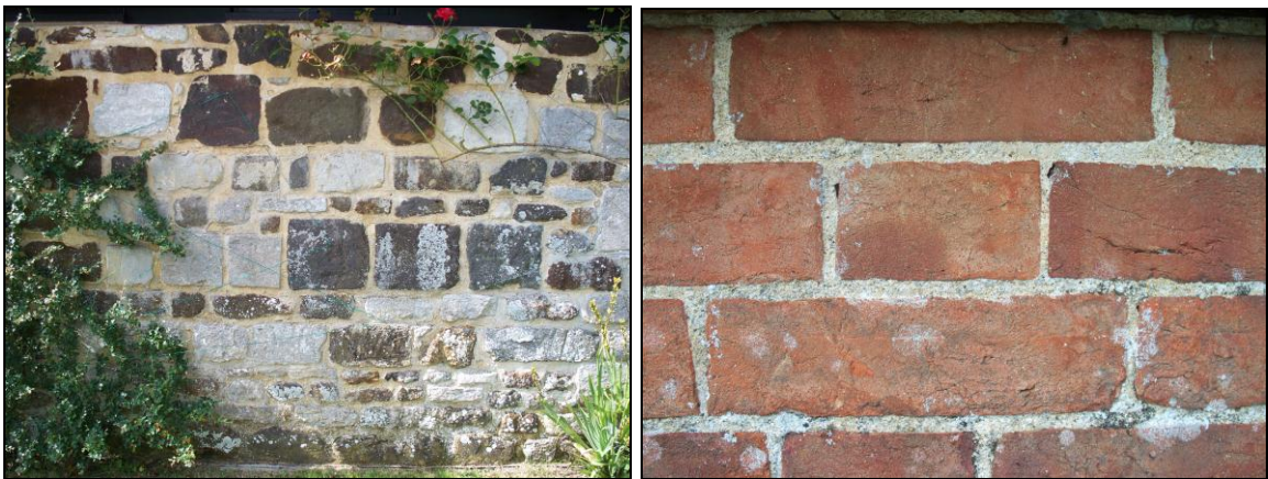
FIG. 10: Walling. Left: Heathstone and limestone masonry seen in the walls of the former barn alongside the Long House. It is likely that this high quality material was salvaged from elsewhere. Right: It is likely that brick seen in the walls of agricultural buildings fronting the main street was manufactured at works historically located just west of the village.
