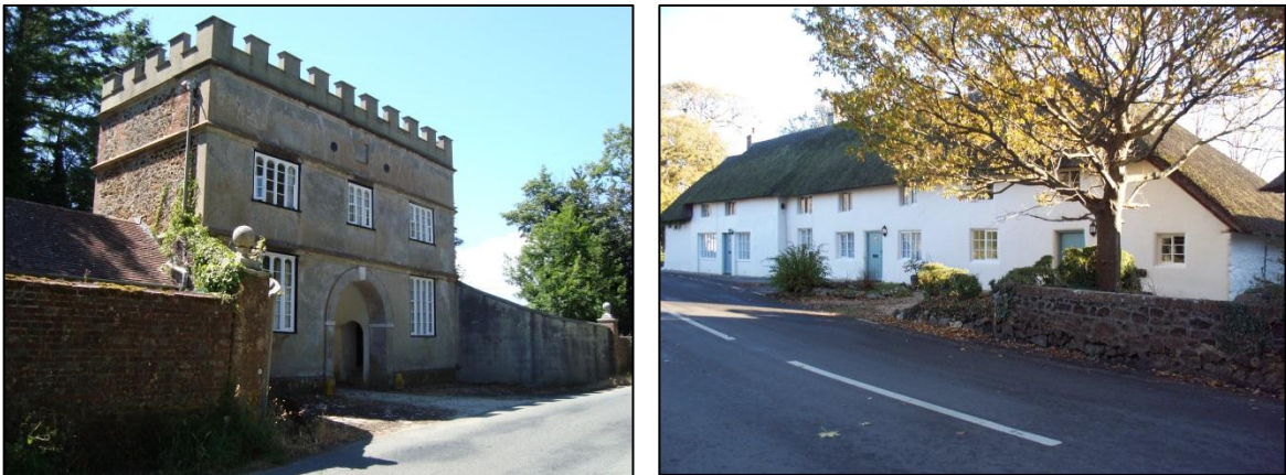
FIG. 13. Render. Wareham Lodge (left) has a flat, formally lined out self-coloured render. This may have been introduced when the structure was moved. Nos. 6-8 (right), which includes the old post office, carries a more informal protective render more typical of the vernacular.
