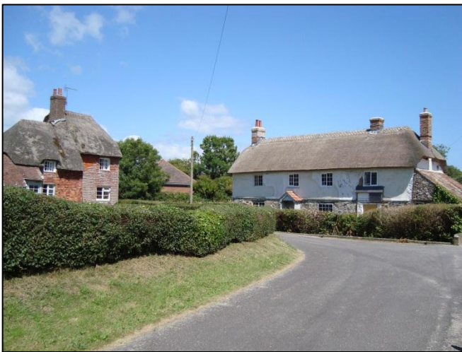
FIG. 14: Cottages at Cockles. No.17 (left) is a visually eccentric building with unusual form and varied palette of materials, including hanging tiles. Nos.18-19 (right) have a more typical form and are constructed from cob on a high rubble stone plinth.
