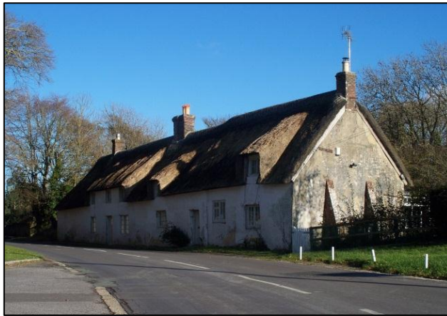
FIG. 15: Nos. 14-16 Main Road. As elsewhere in the village the thatched roof has been renewed. Old photos show a heavy accumulation of what was almost certainly straw thatch, within which the dormers were far less prominent.
