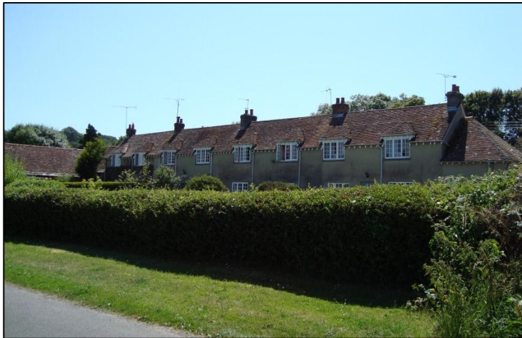
FIG. 16: Nos. 51-54 Shaggs. A distinctive terrace of cottages carrying the date stone 1792.
