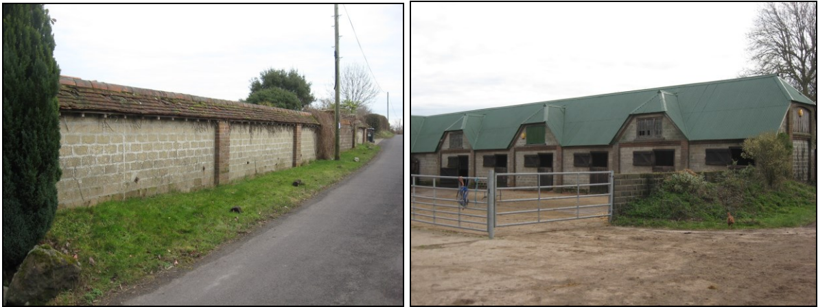
FIG. 21: Bladen Estate blockwork. Estate manufactured block was used in the construction of boundary walls and buildings. Left: boundary wall at Symmond's Barn – note the tiled coping which echoes the weathering provided for cob walls. Modern blockwork is conspicuous where used to fill the former entrance further along. Right: buildings in Affpuddle which again combine block and brick.
