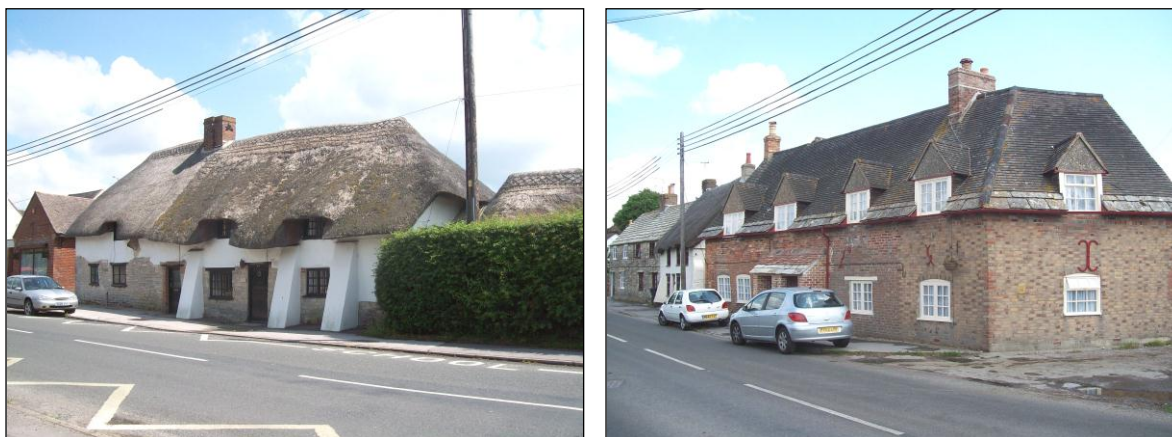
FIG. 2: Eighteenth Century development. Left: Bosun's Cottage. Lower part rubble stone, upper part plastered cob, brick stack, thatched roof with half-dormers and flush ridge. The buttressing is a later addition. Right: Nos. 71 and 73, Corfe Road. Brick with iron tie bars, brick stacks, plain clay tiled roof with stone easing course and half-dormers. Both are listed Grade II.
