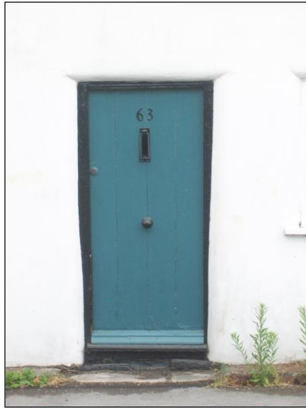
FIG. 11: Door types. Left: traditional plank door at Creech Barrow View. Right: The use of a 'slipped' fanlight is a crude attempt at a Georgian style which erodes quality of character.
