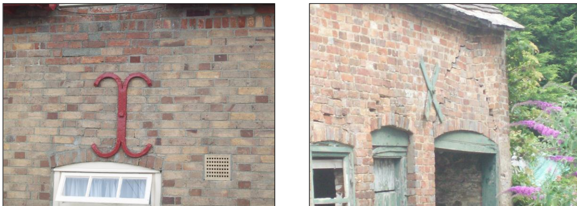
FIG. 8: Pattress plates. Left: No. 73 Corfe Road. Right: Outbuilding serving No. 55 Corfe Road prior to rebuilding work.
