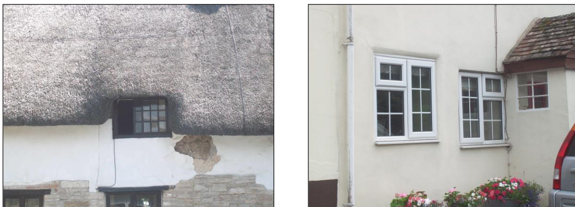
FIG 10: Window types. Left: the sliding sash, shown here on Bosun's Cottage, is a feature traditional to Stoborough. Right: the use of PVC windows has a detrimental affect on the distinctive character of the Conservation Area.
