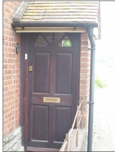
FIG. 11: Door types. Left: traditional plank door at Creech Barrow View. Right: The use of a 'slipped' fanlight is a crude attempt at a Georgian style which erodes quality of character.
