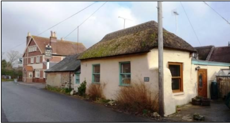
FIG. 17: Converted simple cob outbuildings abutting the High Street, one of which has a thatched roof. Such buildings reinforce the character of this part of the conservation area.
