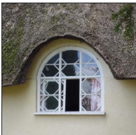
FIG. 14: Windows at Regency Cottage. Note the horizontal sliding sash window.
