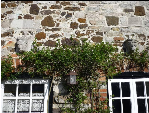
FIG. 12: Corbel heads in front wall of 49 Spring Street.
