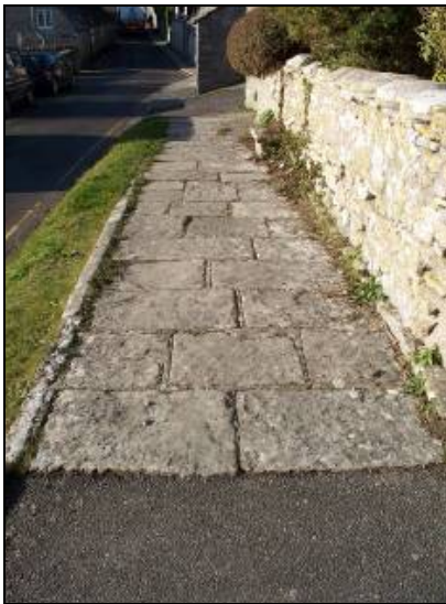
FIG. 7: Stone pavement. An important local feature shared with Conservation Areas in Swanage, Herston, Langton, Kingston and Corfe. Here the pavement has been cut by a tarmac driveway.
