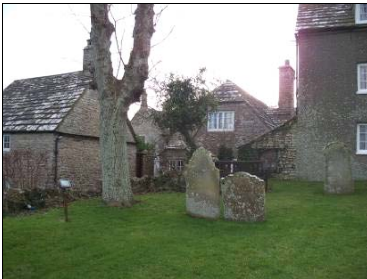
FIG. 4: A cluster of cottages. Formed by Stoneleigh, Lobster Cottage and Church Cottage. Worth House can be seen in the background.
