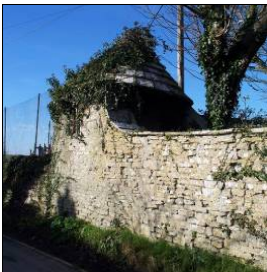
FIG. 10: The gazebo at Worth House.
