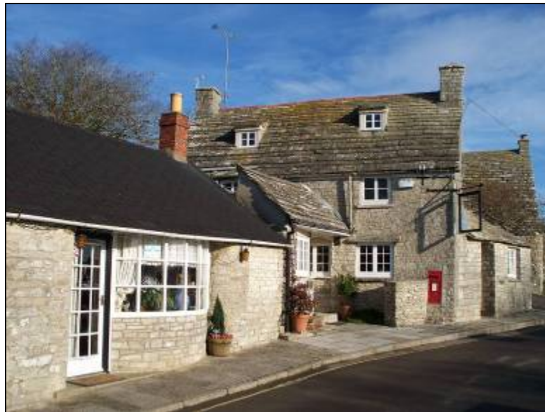
FIG. 2: The café and old post office. The latter has recently closed – note the traditionally proportioned dormers in the roof. Synthetic slate and the clumsy infill between the buildings spoil the scene.
