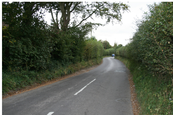
6. Fairmile Road looking south.
