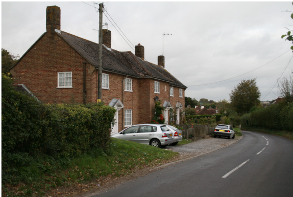
7. Fairmile Road looking north, with Lower Bryanston Cottages to the left.
