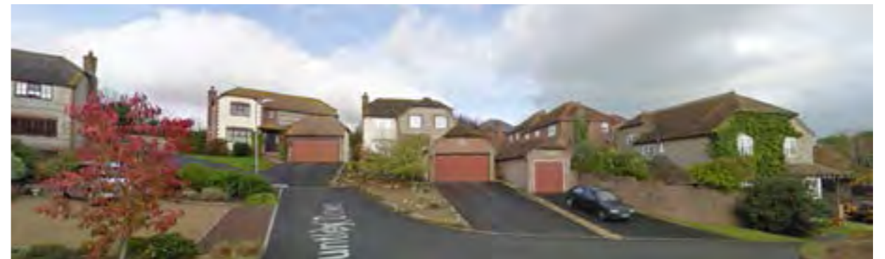
3.0 View of the sloping site and how garages have been designed accordingly
