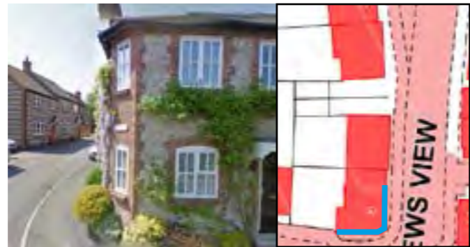
St. Andrews View. Red brick and stone corner building
