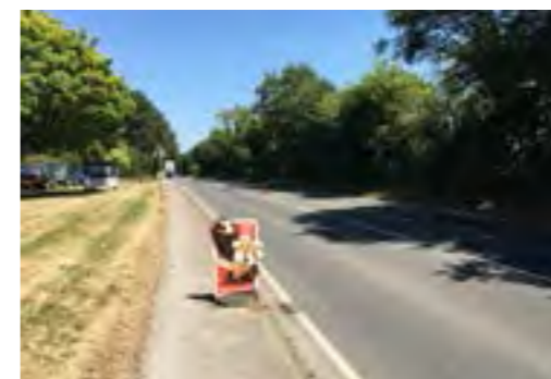
5.0 A354 Looking East
