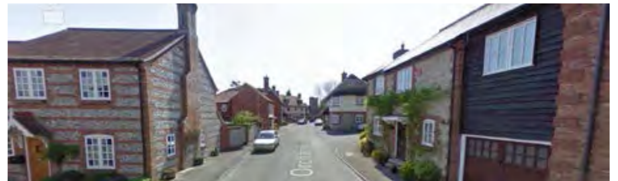
2.0 View of St. Andrews view
