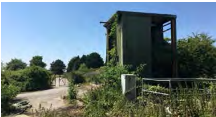
3.0 Disused industrial buildings
