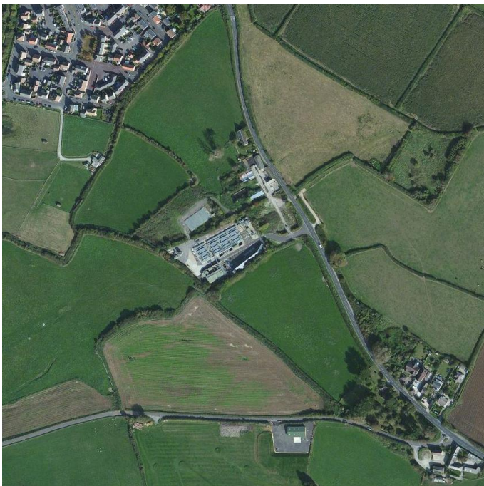
Figure 3c: Bridport Sewage Treatment Works
