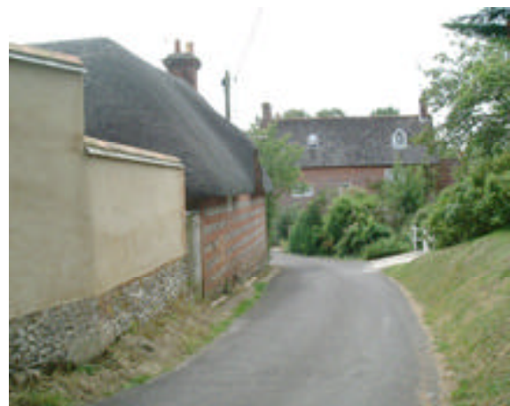
Boundary wall adjacent to Sinodun in Grugs Lane
