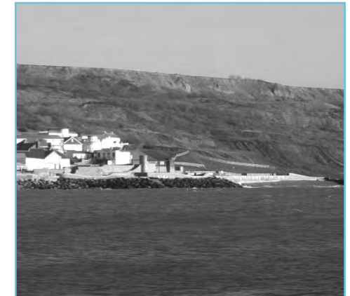
Phase IV of the Coastal Protection Scheme
