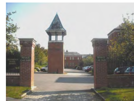
Fig 31 Main entrance to Greenwood House
