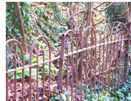
Fig 30 Hoop railings of Herrison House
