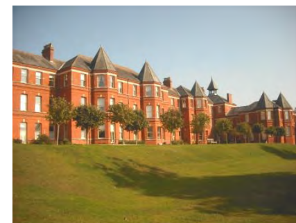
Fig 18 Southerly side of Greenwood House
