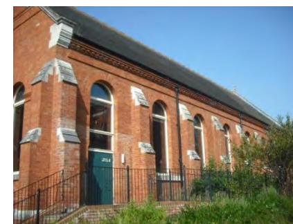
Fig 21 East elevation of Herrison Hall
