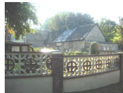
Fig 26 Garden wall of No 13 Herrison Rd & attached farm buildings
