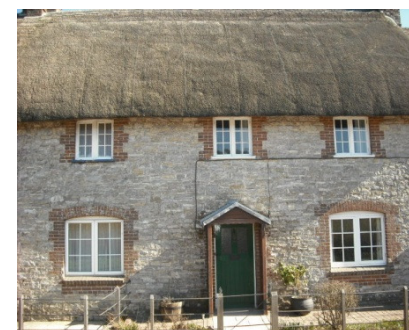
Fig. 15 No 2 Rectory Cottages
