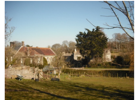
Fig. 7 View of The Old Rectory & Warmwell House from the churchyard
