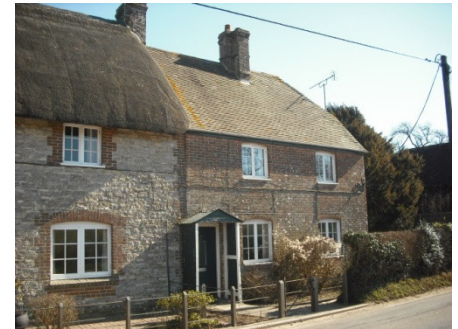
Fig. 5 No 1 Rectory Cottages
