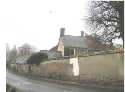
Fig. 11 The Old Rectory & boundary wall
