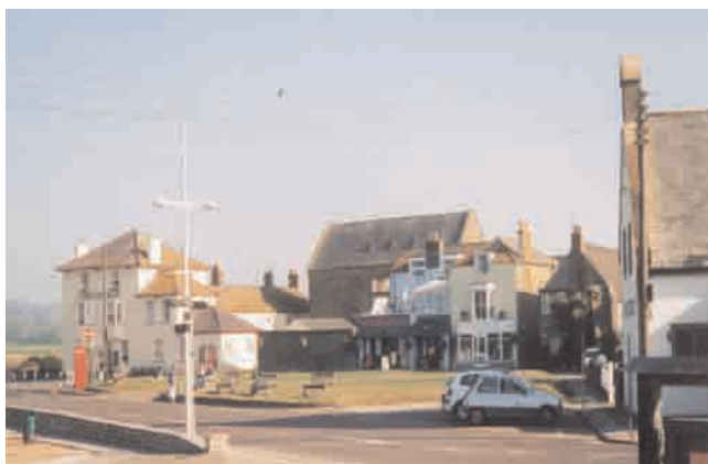
Fig 10. View northwards towards Harbour Green.
