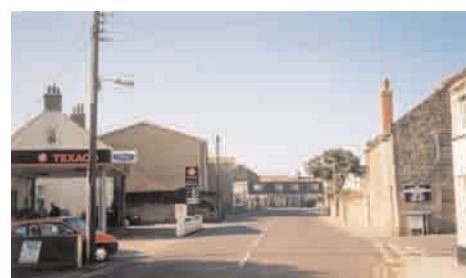
Fig 52. West Bay Road near Harbour Garage.
