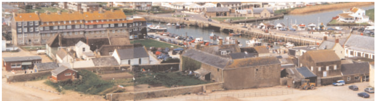
Fig 39. View from East Cliff with the Shared Garden & Messrs Norman Good's former Bonded Stores in the foreground.
