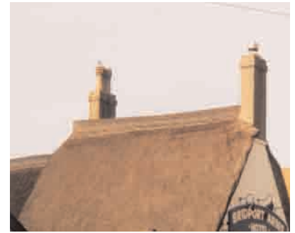
Fig. 17. Laced thatch ridges.
