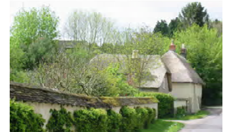
Roofing materials, Piddlehinton
