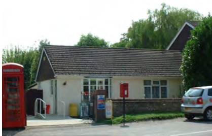
The former Piddlehinton village shop
