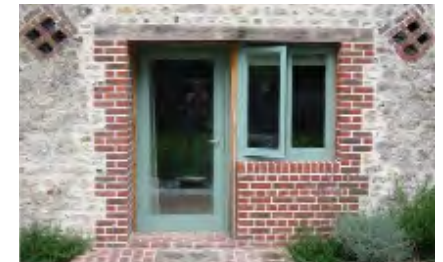
Replacement doors and windows, Plush
