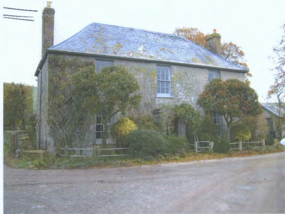
FIGURE VIII: GOURDS FARMHOUSE (FORMER MANOR FARM)
