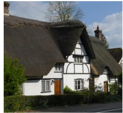
Former Inn C15
