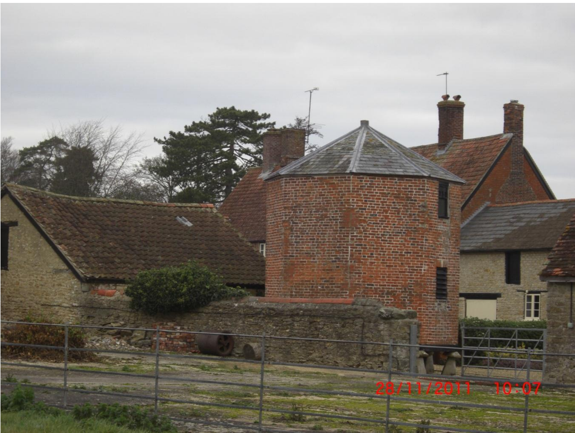
Wyke Farm outbuildings with the brick granary centre.
