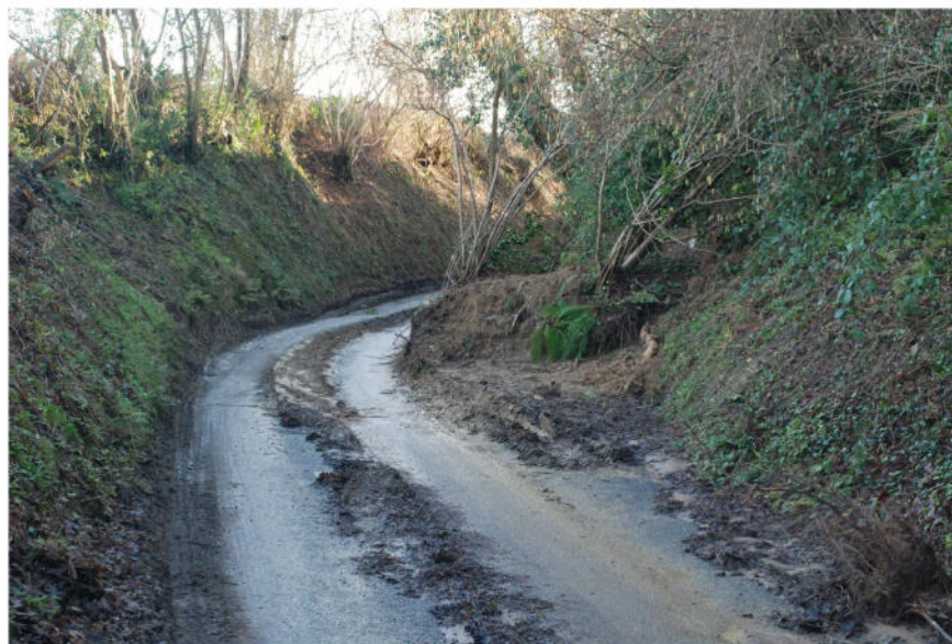
Fig. 7. Landslip in sunken lane, Stedham, West Sussex.
