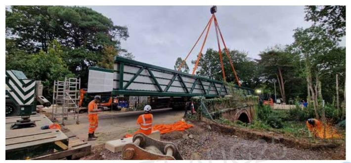
New active travel bridge being installed next to the road bridge over the railway line in Glenferness Avenue Bournemouth as part of Transforming Travel corridor.
